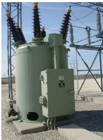
a) 66 kV Oil Circuit Breaker
